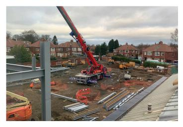
With foundation works now completed on our North End Development, principal contractor Tolent has begun erecting the steel frame.
